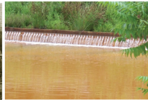
Abandoned mine drainage flows through the treatment ponds.
