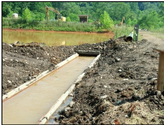
New trough installed between the first and second ponds at Lowber.
