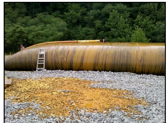
Geotube being filled with iron sludge.
