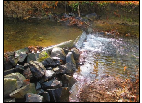
This jack dam was repaired to control erosion of the nearby stream banks and add oxygen to the water.
